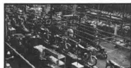
The plant is at full capacity for production increase.
