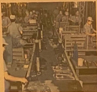
▲ "Casing assembly: minute parts are assembled with scrupulous cares."
