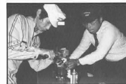
A torque wrench is used to assemble a con-rod.
