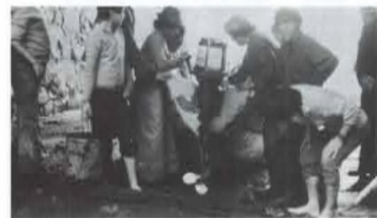
Boat transom is cut a little for better fitting a motor.
