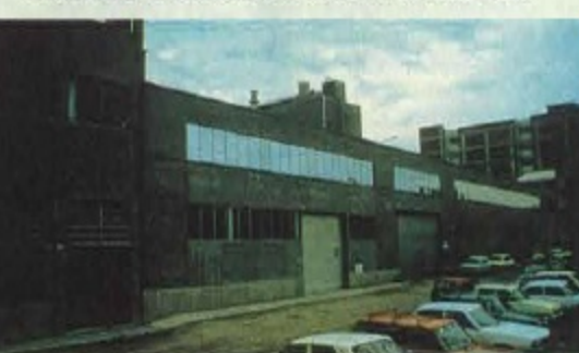
SEMSA's factory building
