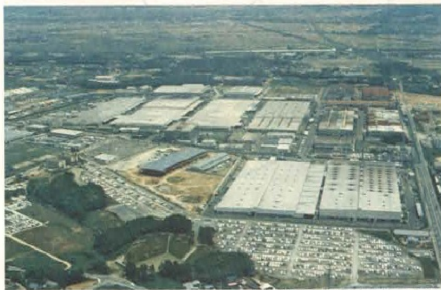
Main office and factory buildings at Iwata
