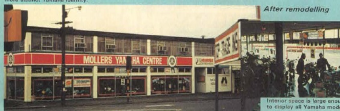
Mollers Yamaha Center - Auckland Auckland is the largest regional market in this country. Mollers Yamaha's branch shop which covers this important market is also redesigned. Red stripe is effectively used for more distinct Yamaha identity.
