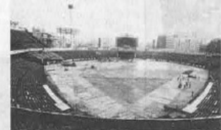
Plastic sheets were laid out all over the artificial turf of the stadium grounds. Next, 7,500 boards carried in place by forklifts were laid out on what was to be the track. After this, the ground was covered once more with plastic sheets. This was a precaution to make sure that the artificial turf would not get covered with dirt even if it rained and began to wash away.
