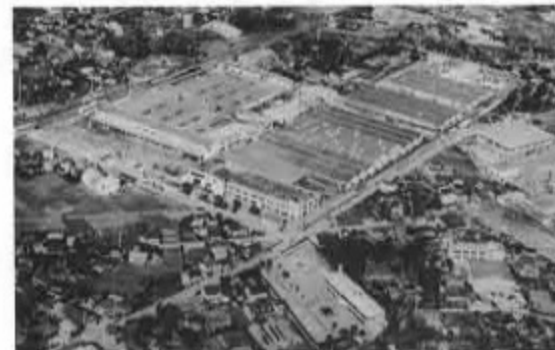
An aeroplane view of the plant
