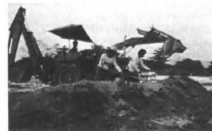
A bulldozer and shovel loader are used to make up a training course.
